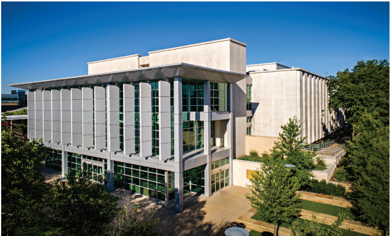
The renovators of the interior discovered that the Founders Building had been built to top-of-the-line standards in 1964. The three-story addition to the east end of the original building provided sidewalk-level access to the building from the center of campus as well as study and congregation spaces.
