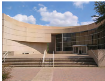
Uninviting building entrance
