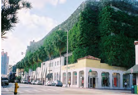
Parking structure fit into the urban context
