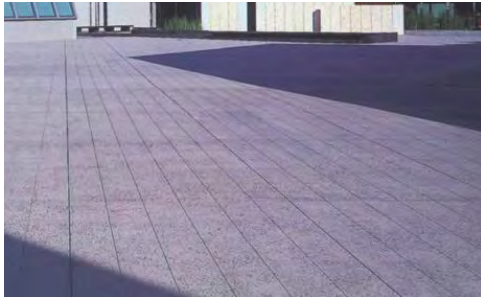
Saw cut concrete
