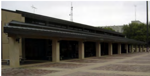
Existing colonnade along Student Union
