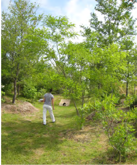
Drainage channel at University Parkway at the current mock up
