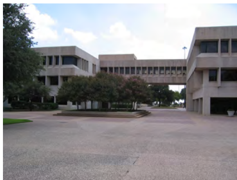
Skywalks connecting the buildings
